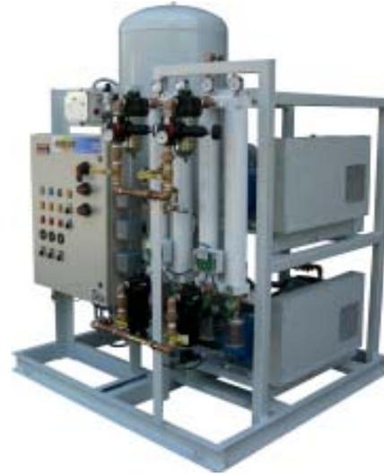
The dryer is designed to provide a maximum dew point below +32°F per NFPA 99. Built-in purge saver control automatically minimizes the amount of purge air to match the variable air flow. Each dryer is equipped with a 0.5 micron pre-filter with electronic drain and element change indicator, 0.5 micron after-filter with element change indicator and a pressure regulator.
